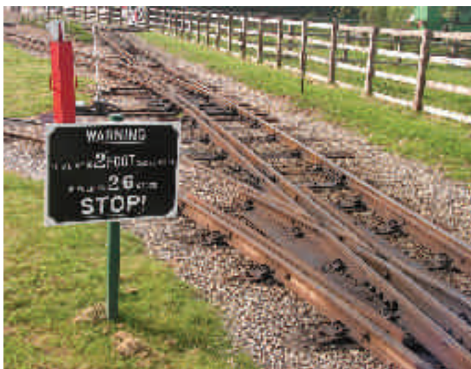
Photo 3. Flat crossing - 2ft / 2ft 6in dual gauge line over standard gauge.
