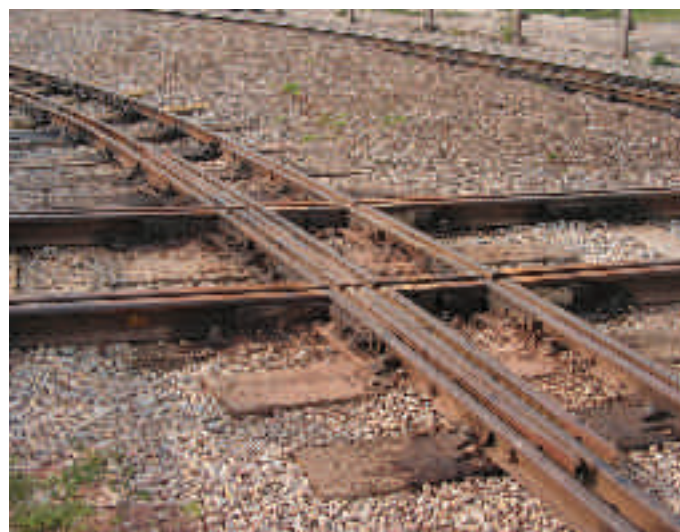
Photo 3. Flat crossing - 2ft / 2ft 6in dual gauge line over standard gauge.
