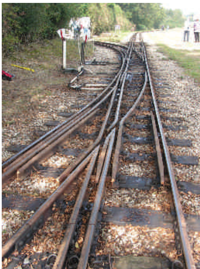
Photo 2. 2ft / 2ft 6in gauge pointwork at Oak Tree Halt.
